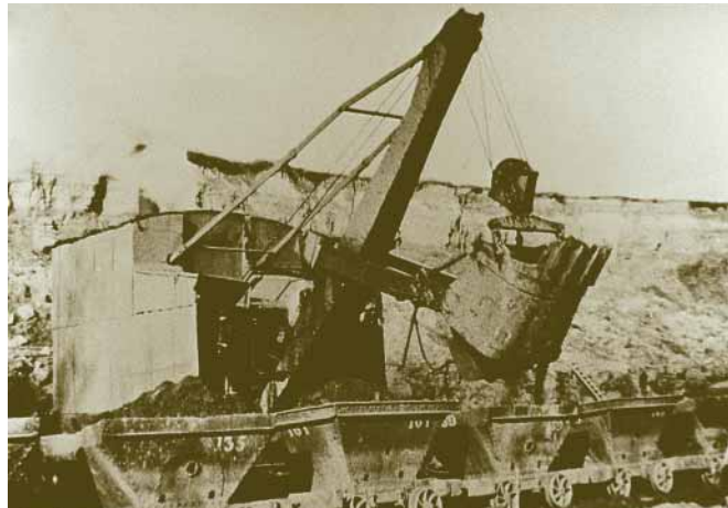
Ruston 20 ton steam shovel loading ore.
